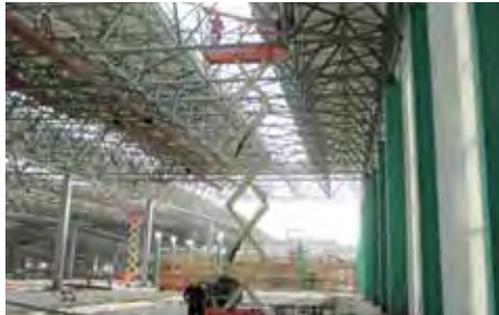
China: Check on construction sites
